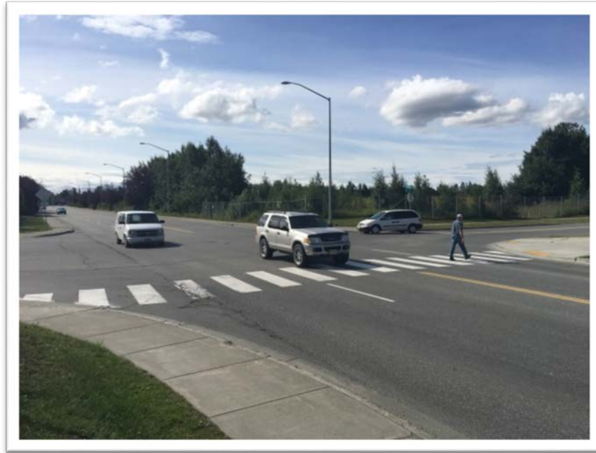
FIGURE 3. DENALI STREET AND 40 TH AVENUE INTERSECTION, LOOKING SOUTH
