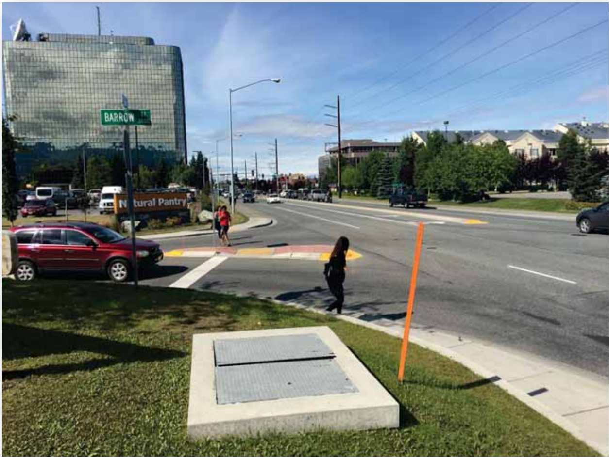
Figure 57: ACS Vault on 36 th Avenue
