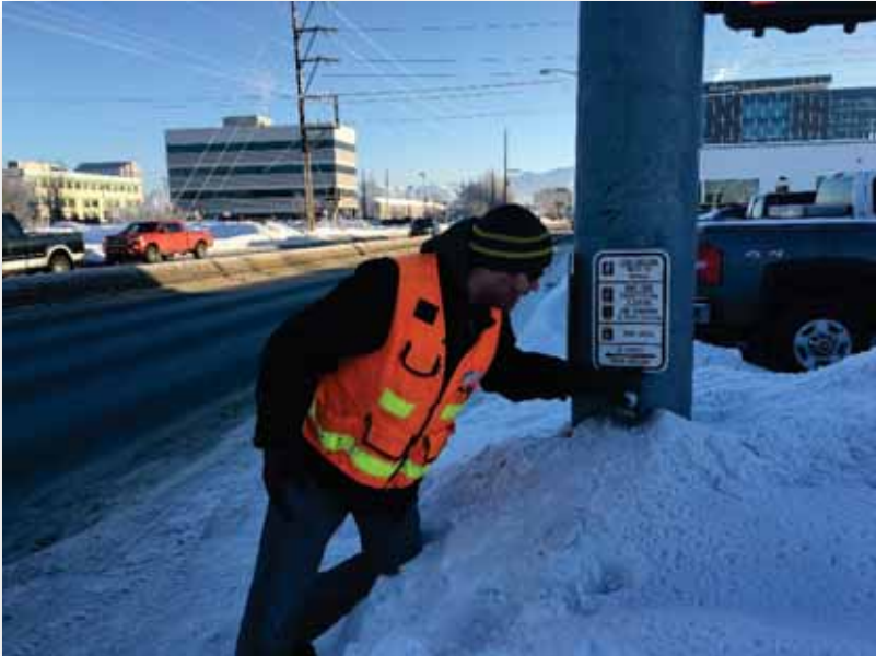
Figure 59: Snow restricting access to pedestrian push button
