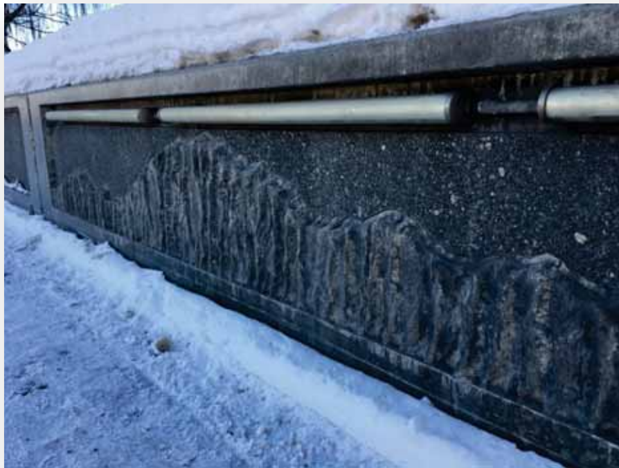
Figure 10: Decorative landscaping wall along Denali Street
