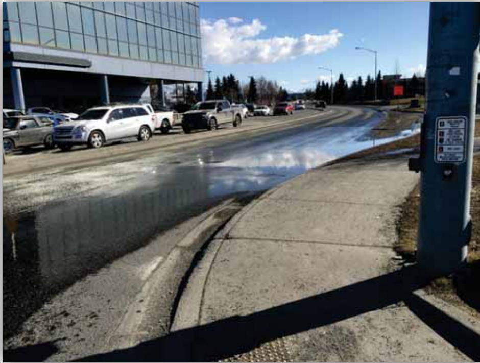
Figure 55: Ponding on Denali Street south of 36 th Avenue
